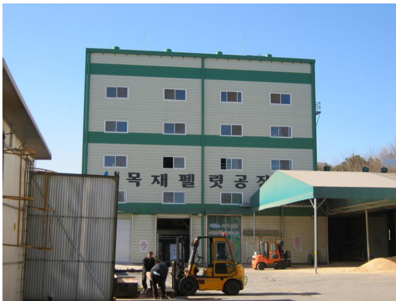
Figure 4. Pellet plant with lumber drying kiln in left foreground
