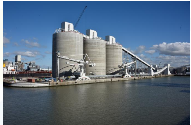
Biomass discharge berth / CSUs - Liverpool
