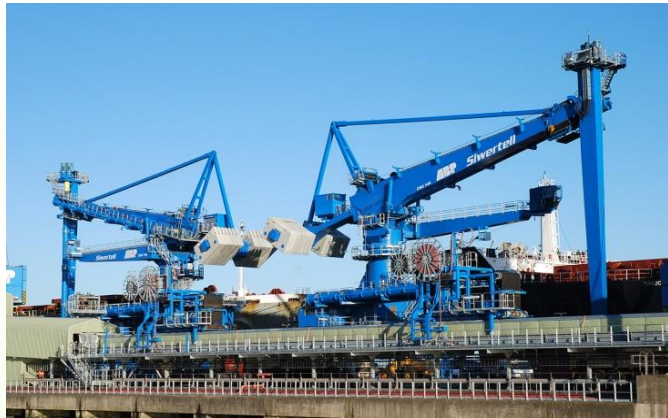
Siwertell CSU – image prior to incident
